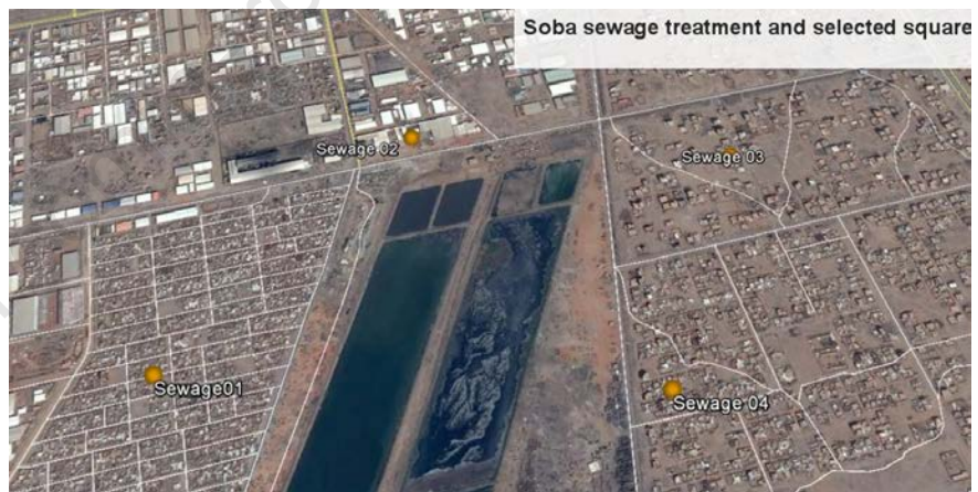
Figure 2. Selection of squares mostly affected by Soba sewage treatment plant.
