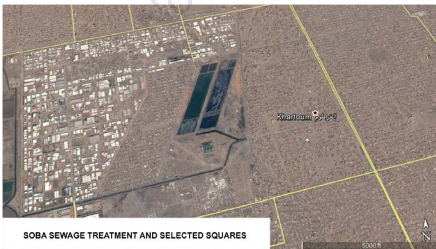
Figure 1. Soba sewage treatment plant.
